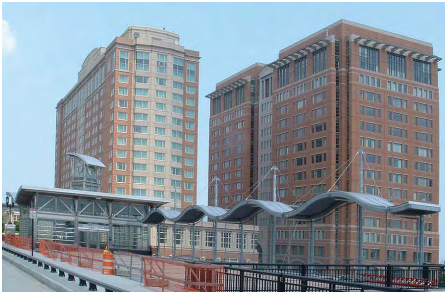
A tripartite agreement among the MBTA, Massport, and a developer in South Boston led to construction of a new underground Silver Line BRT station.
