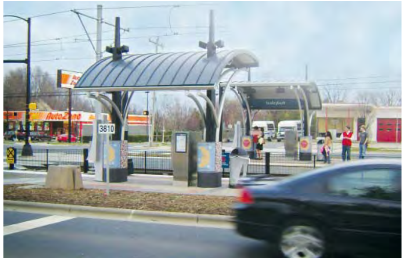
The City of Charlotte purchased property at Scaleybark station, which is surrounded by large industrial and commercial sites, to ensure that development remains affordable.
