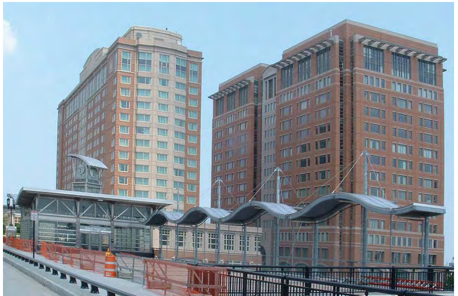
A tripartite agreement among the MBTA, Massport, and a developer in South Boston led to construction of a new underground Silver Line BRT station.
